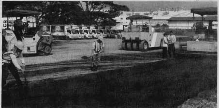
File photo provided by SMC when it started testing asphalt produced with recycled plastic waste and bitumen on a 1,500 sqm pilot site at its new logistics center in General Trias, Cavite.
